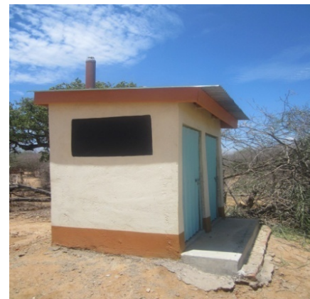
Sanitation facility - latrine
