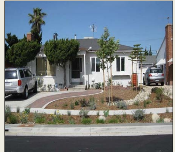
Elmer Avenue Retrofit
