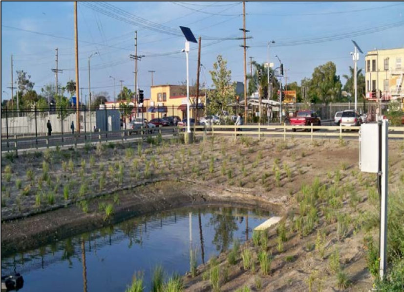
Wetland Cell Construction
