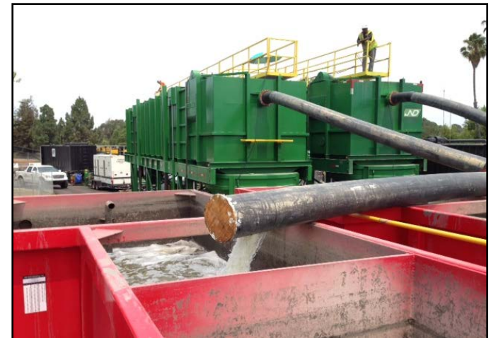
Sediment Dewatering Return Water
