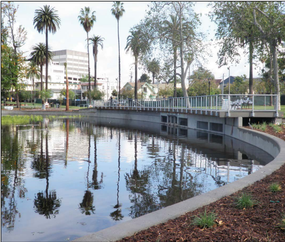
Stormwater Inlet to the Lake
