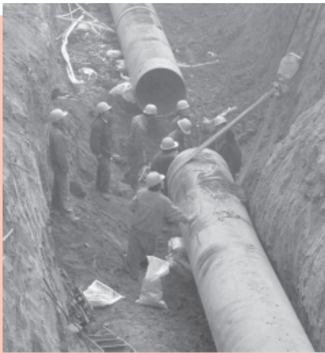
West East pipeline construction
