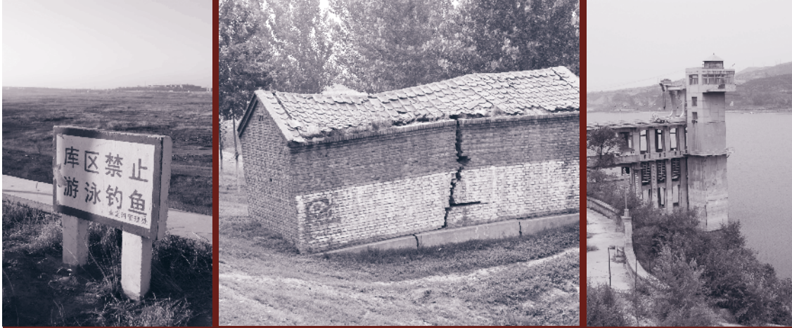
1-No Fishing or Swimming sign on the “bank” of Daning reservoir.; 2-Building in the outskirts of Beijing destroyed due to settling caused by falling water table.; 3-Guanting Reservoir now holds only a fraction of its capacity. Photo credit: Wang Jian.
